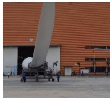
Previous blade installation method by forklift and transfer fixture
